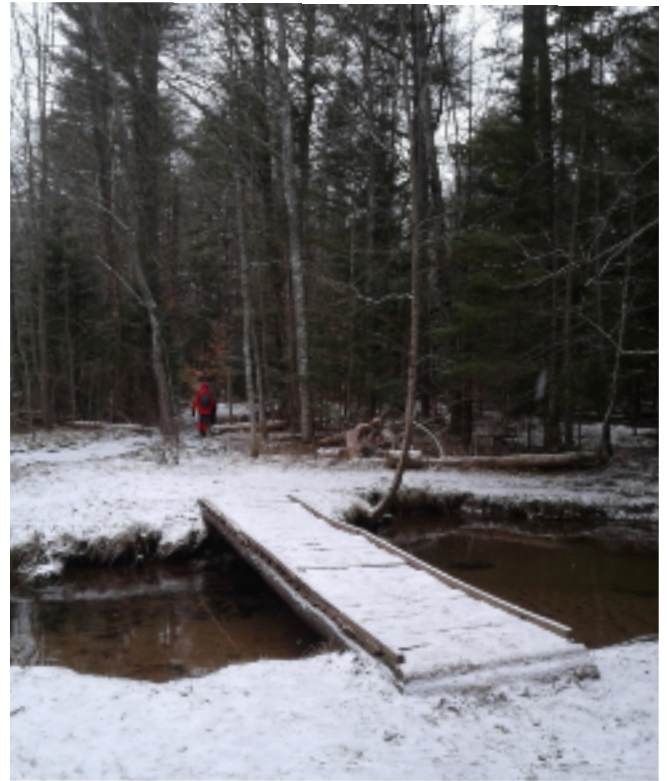
Bridge over Spidle Brook.
